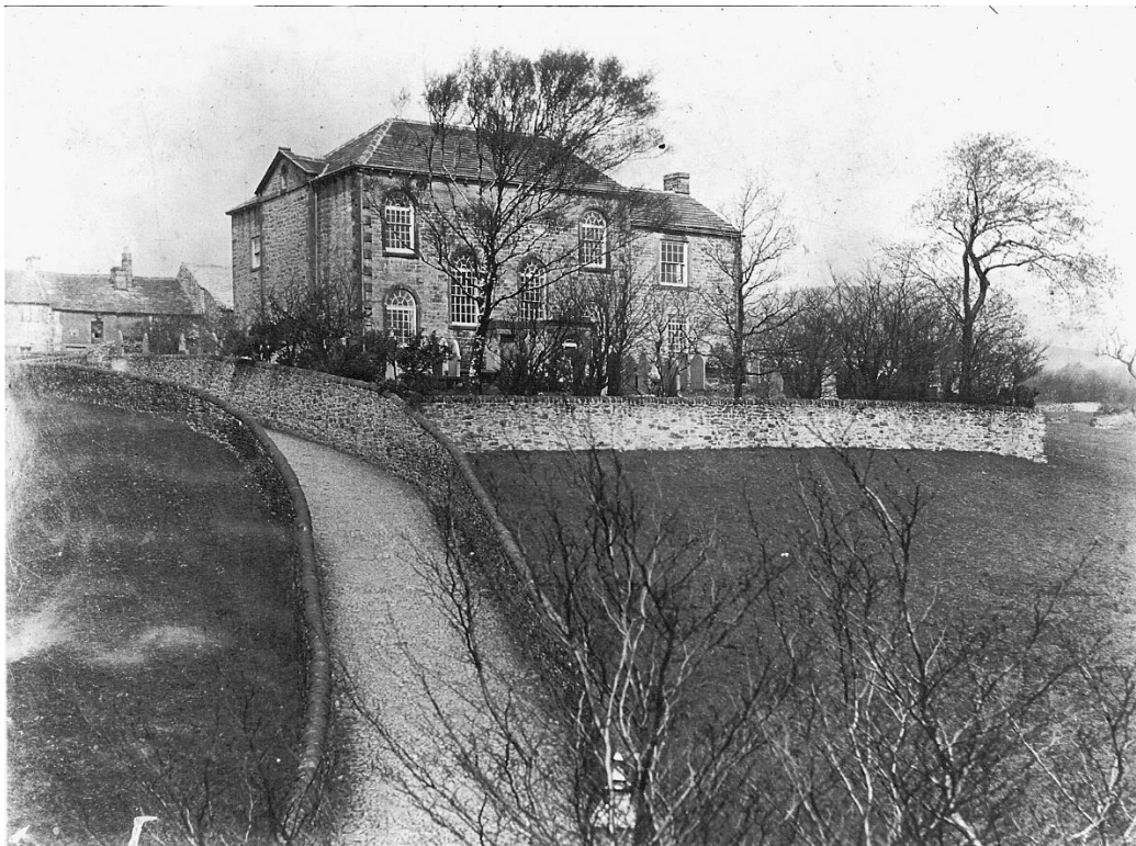
The original chapel and access road from the south
